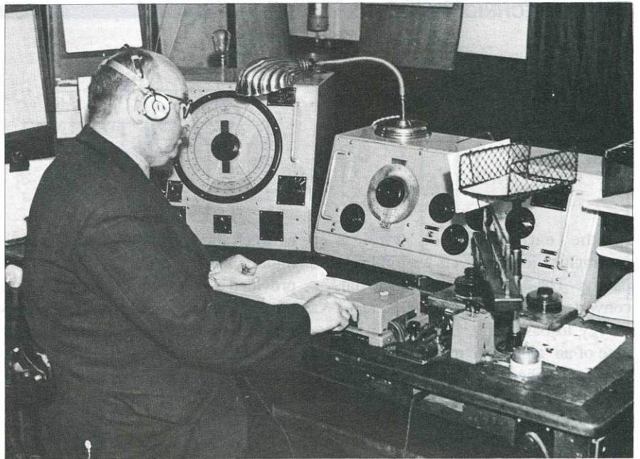
Fig. 5 - Post Office receiver and goniometer No. 7
